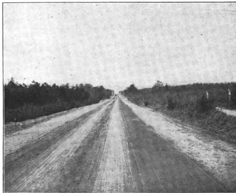
CORLISS AVENUE AFTER IMPROVEMENT—A FINE STRAIGHTAWAY STRETCH.
